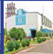
Orion Power Meghnaghat Ltd.
