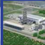
Orion Power Sonargaon Ltd.
