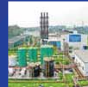
Dutch Bangla Power & Associates Ltd.
