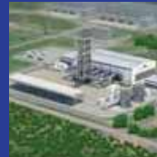
Orion Power Sonargaon Ltd.
