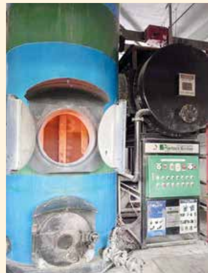
Existing biomass boiler fuelled by Jhut (waste fabric), which is neither environmentally friendly nor aligned with circular economy principles.
