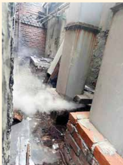
Current state: Condensate used in the dryer and ironing stations is being released into the air in a washing and printing factory.
