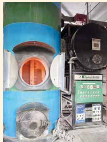
Existing biomass boiler fuelled by Jhut (waste fabric), which is neither environmentally friendly nor aligned with circular economy principles.
