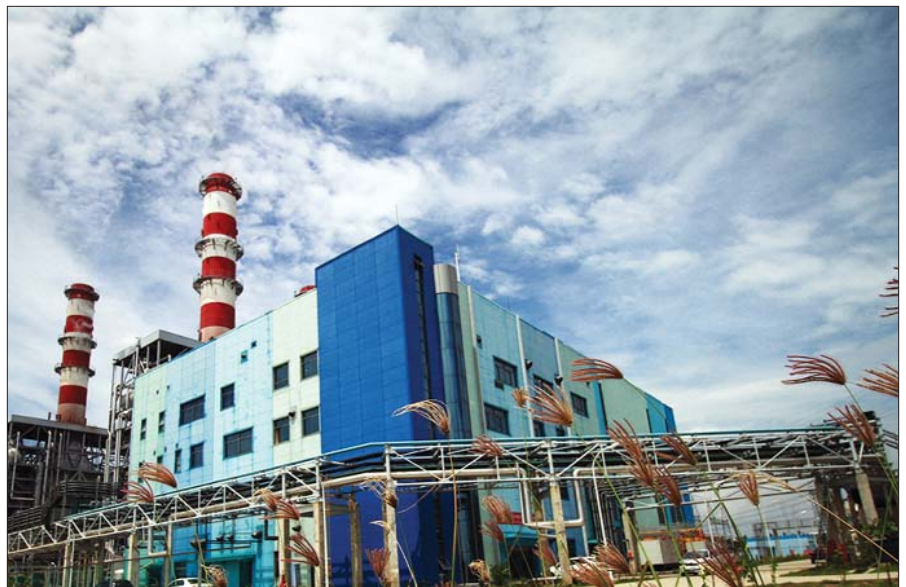
Summit Meghnaghat Power Plant
