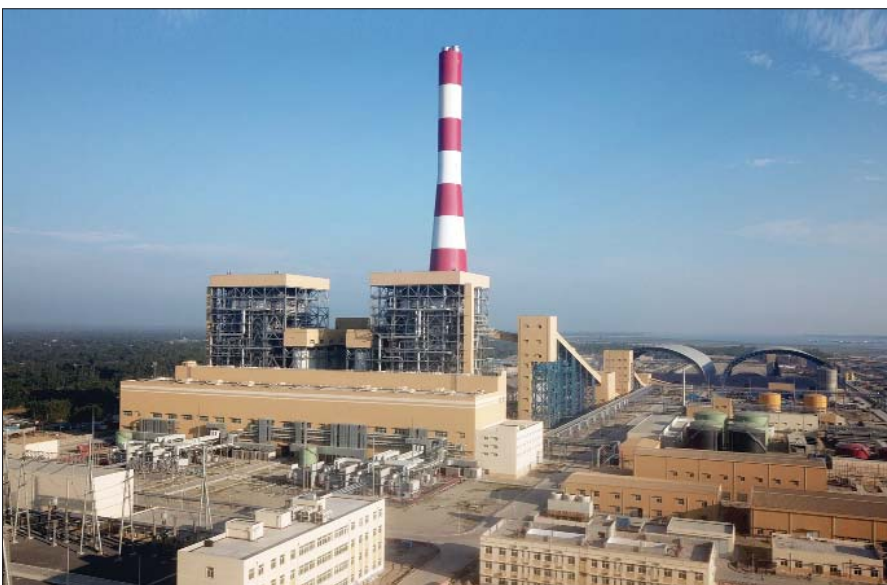
1200 MW SS Power Coal Based Power Plant in Chattogram
