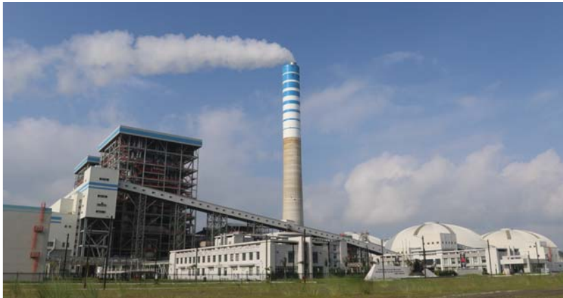
1 st Ultra-Supercritical Power Plant of Bangladesh
