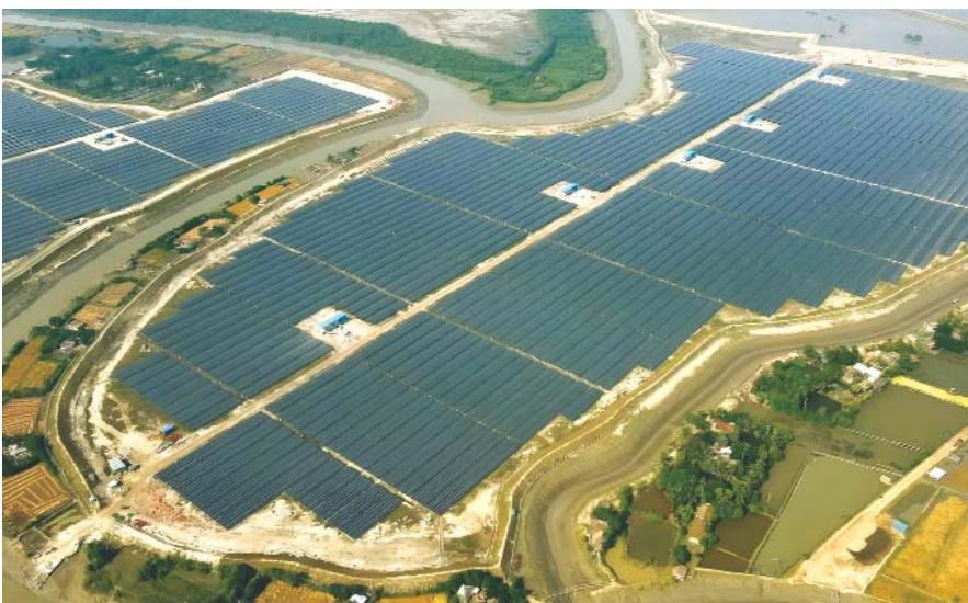
A view of a 200MW Teesta Solar Plant
