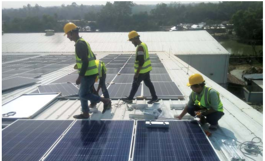
A view of an under-construction solar rooftop project
