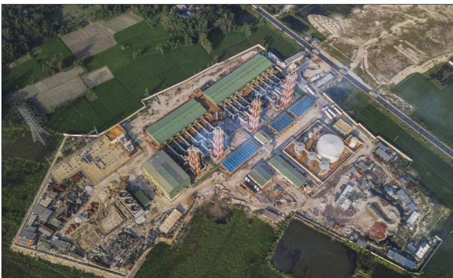
Liquid fuel-based power plant of Confidence Group in Rangpur
