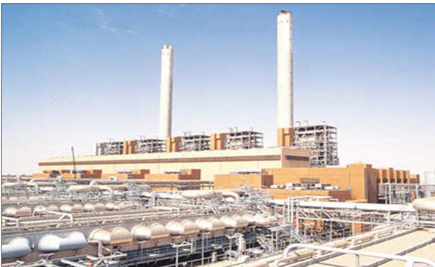
A combined-cycle Unique Meghna Ghat power plant is ready for electricity generation but necessary gas supply is yet to be assured
