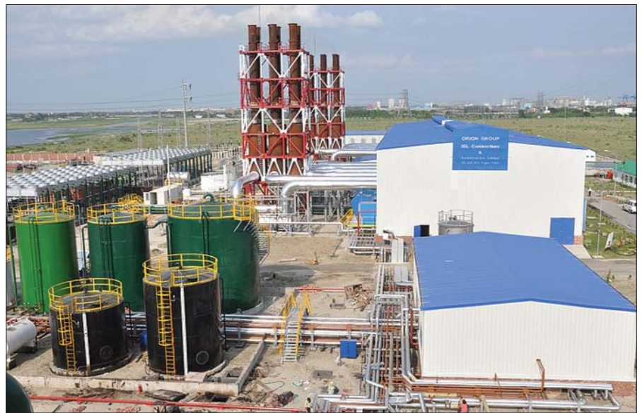
HFO-based power plant of Orion Group at Meghna Ghat
