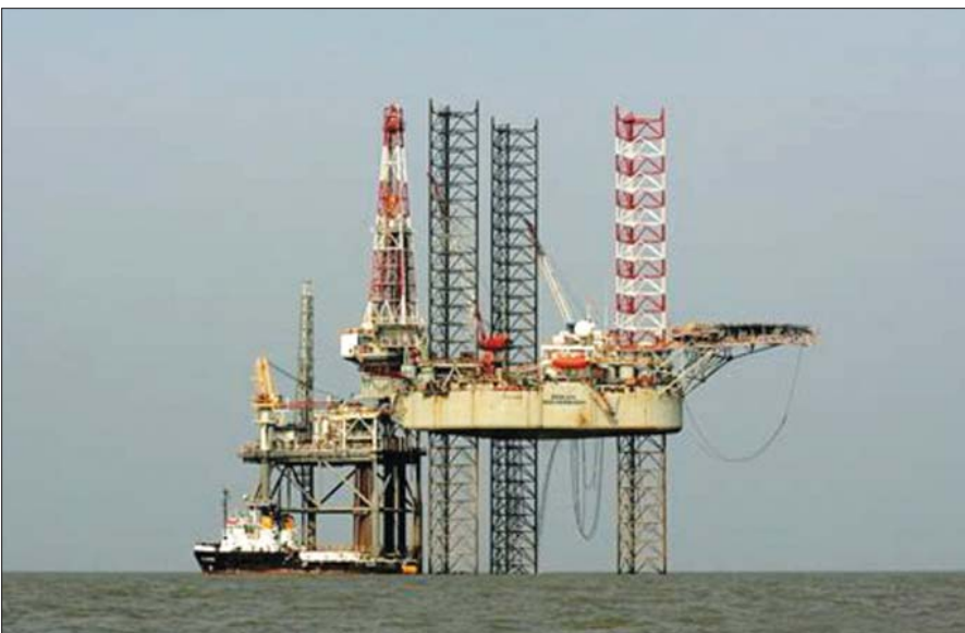
Abandoned offshore gas field at Sangu
