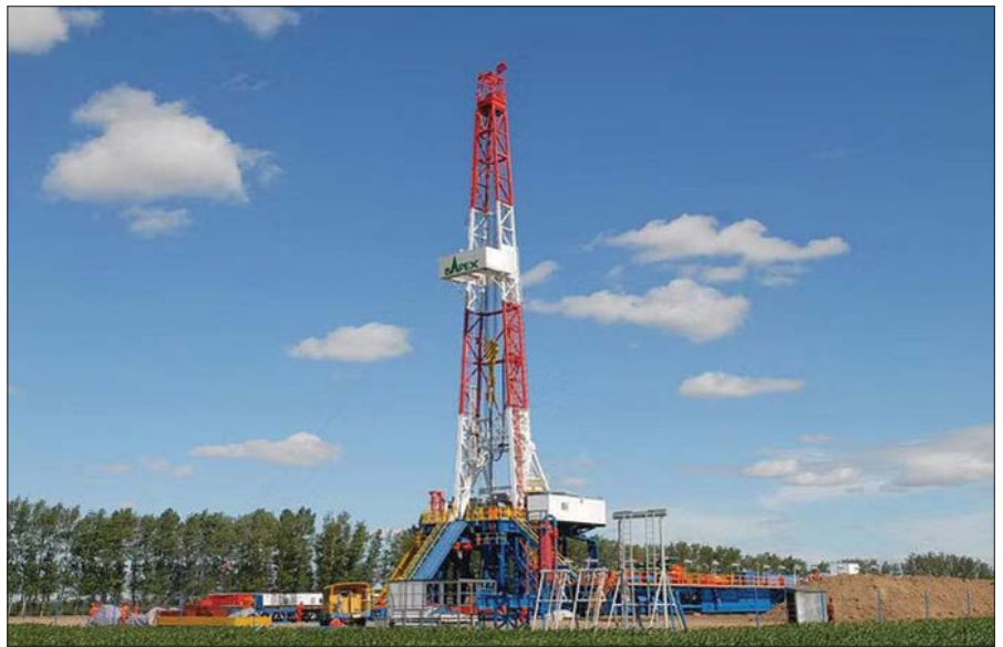
A view of BAPEX's exploration drilling rig working at a field in Bangladesh
