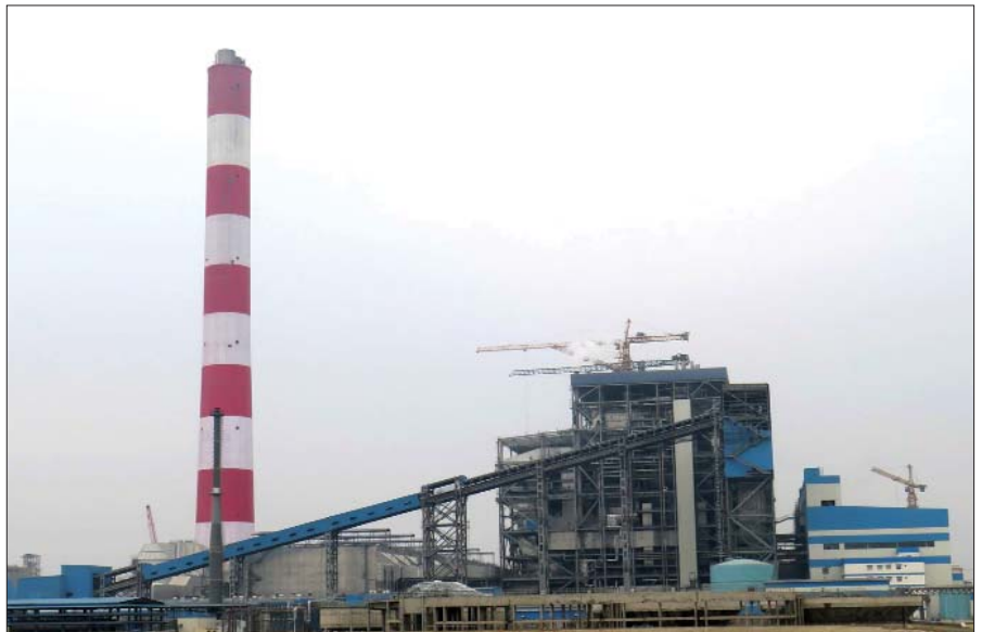
Adani's 1600MW coal-based Godda Power Plant
