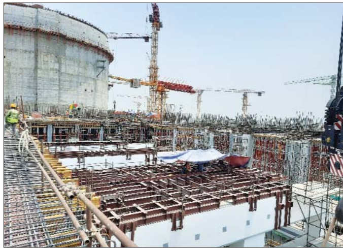
Temporary Steel Support Installation
