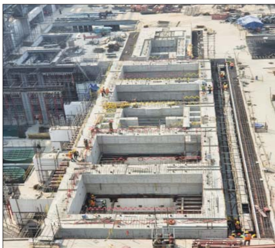
TG Deck after 1st stage of concreting
