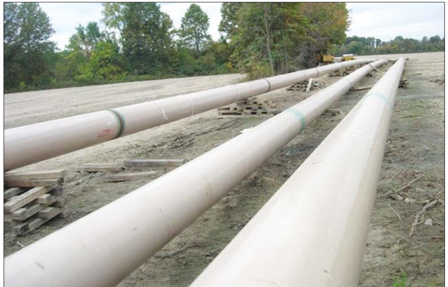
View of a under construction gas pipeline
