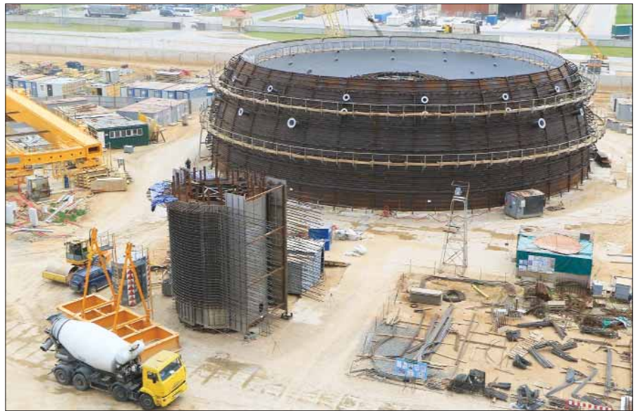
RNPP construction work in progress
