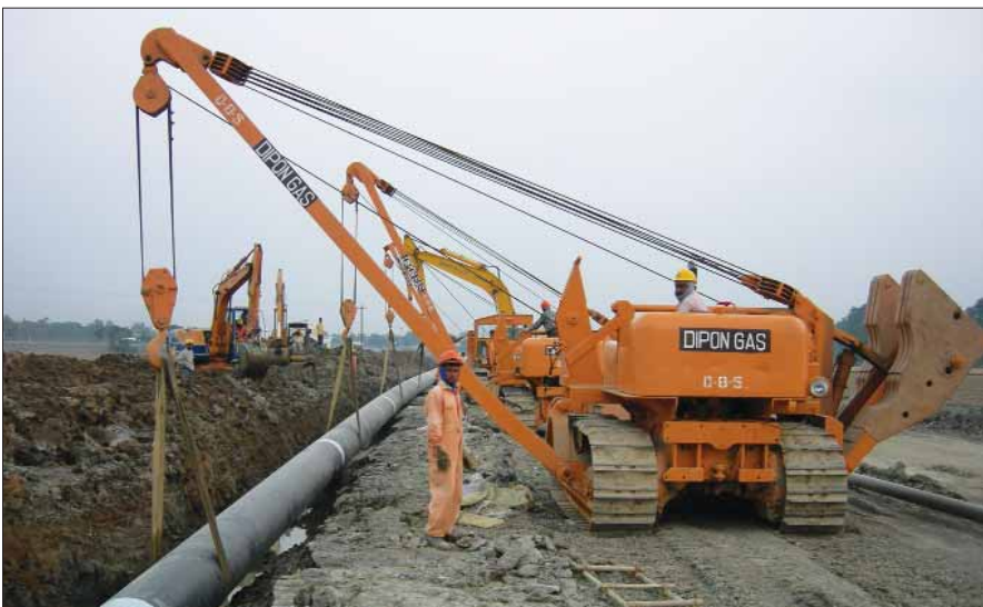
Gas transmission pipeline work in progress
