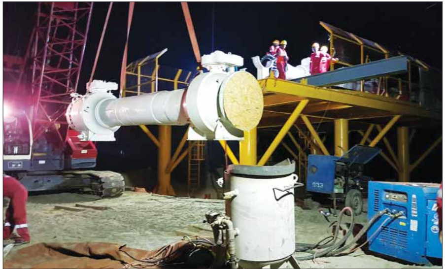
Gas transmission pipeline work in progress
