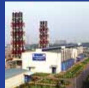
Digital Power & Associates Ltd.
