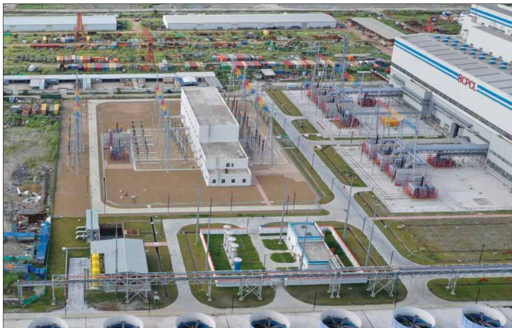
Payra 1320MW Power Plant
