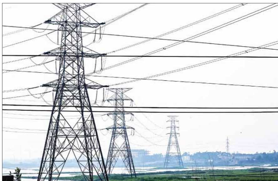
Power Transmission Tower
