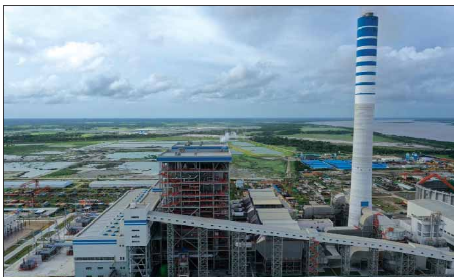
A view of Payra 1320MW Power Plant
