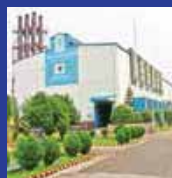
Orion Power Meghnaghat Ltd.
