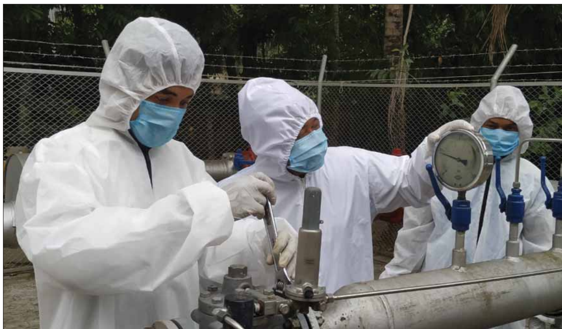
GTCL workers doing regular maintenance work at a City Gate Station
