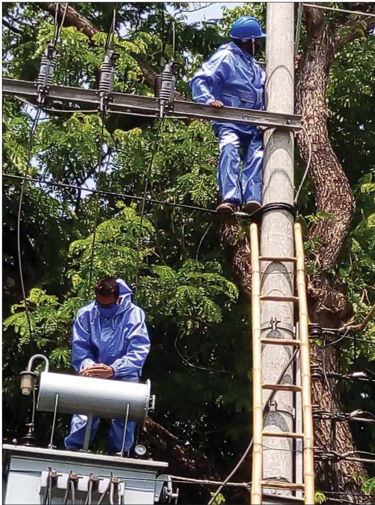
REB line maintenance work during COVID-19 pandemic period
