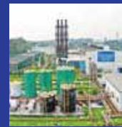
Dutch Bangla Power & Associates Ltd.
