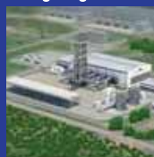
Orion Power Sonargaon Ltd.
