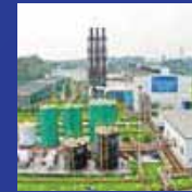
Dutch Bangla Power & Associates Ltd.
