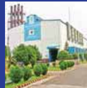
Orion Power Meghnaghat Ltd.
